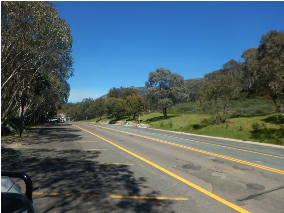
Figure 9: View from Friday Drive headed towards the village
