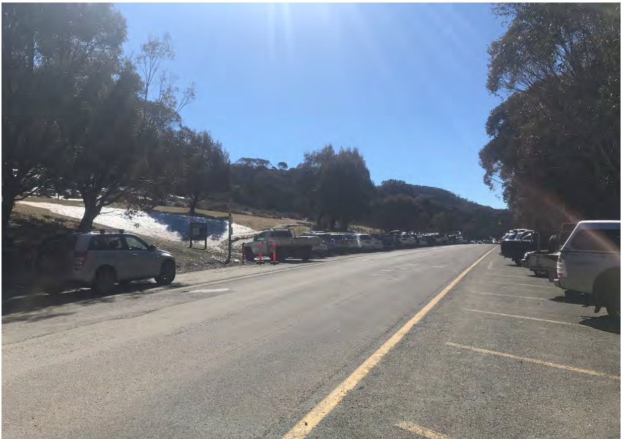
Photo 4: The approximate location of the proposed on ramp at the southern end of the proposed car park.
