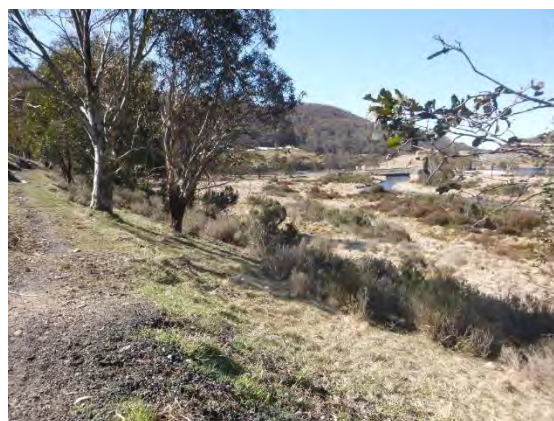
Plate 2: view north east along Thredbo River flats to carpark 3 location showing constructed bank to carpark
